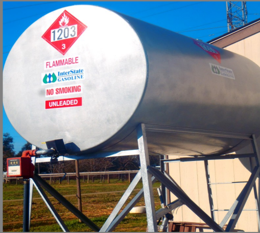
550 gallon tank on stand
