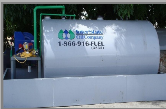
2,000 gallon double walled tank in containment
